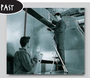
HVAC engineers and technicians work together to measure volume flow. The engineer relays the required grid measurements to the technician who enters the data from the numerous measuring points by hand into a manual datasheet.
